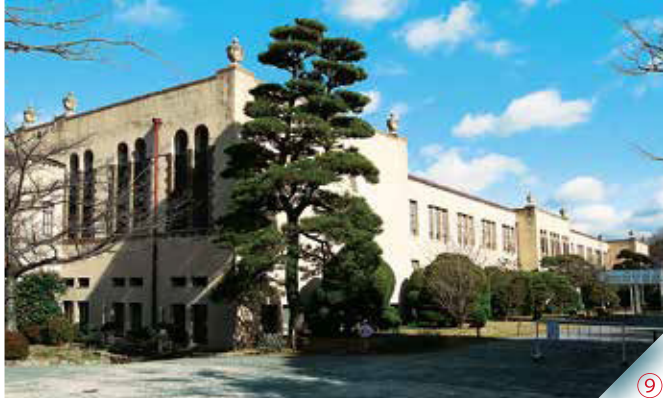
葆光館(中高部) Hokokan(Academy Building)
