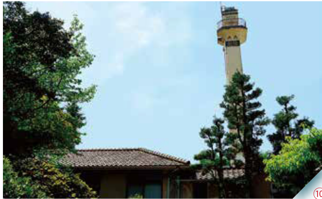
汽罐室と煙突 Power House of Dormitory Section
